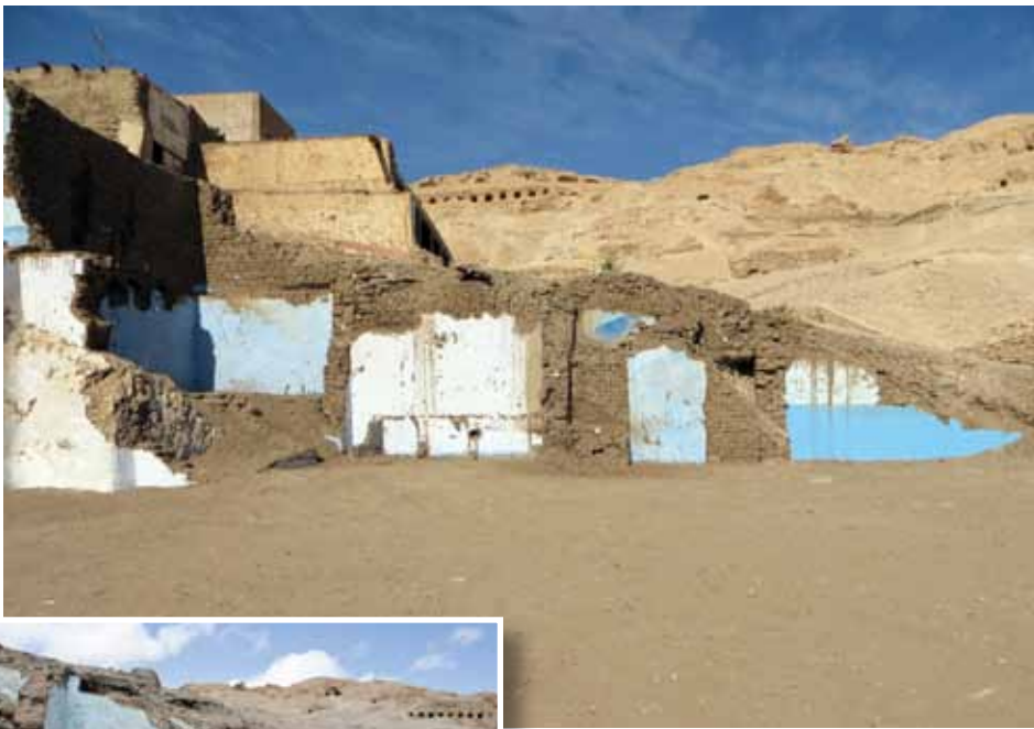
LEFT One of the largest buildings at el-Qurna was accommodation rather alarmingly called 'Snake Motel'. INSET Burial chambers were often used as bathrooms, like that seen here in section Q05.
